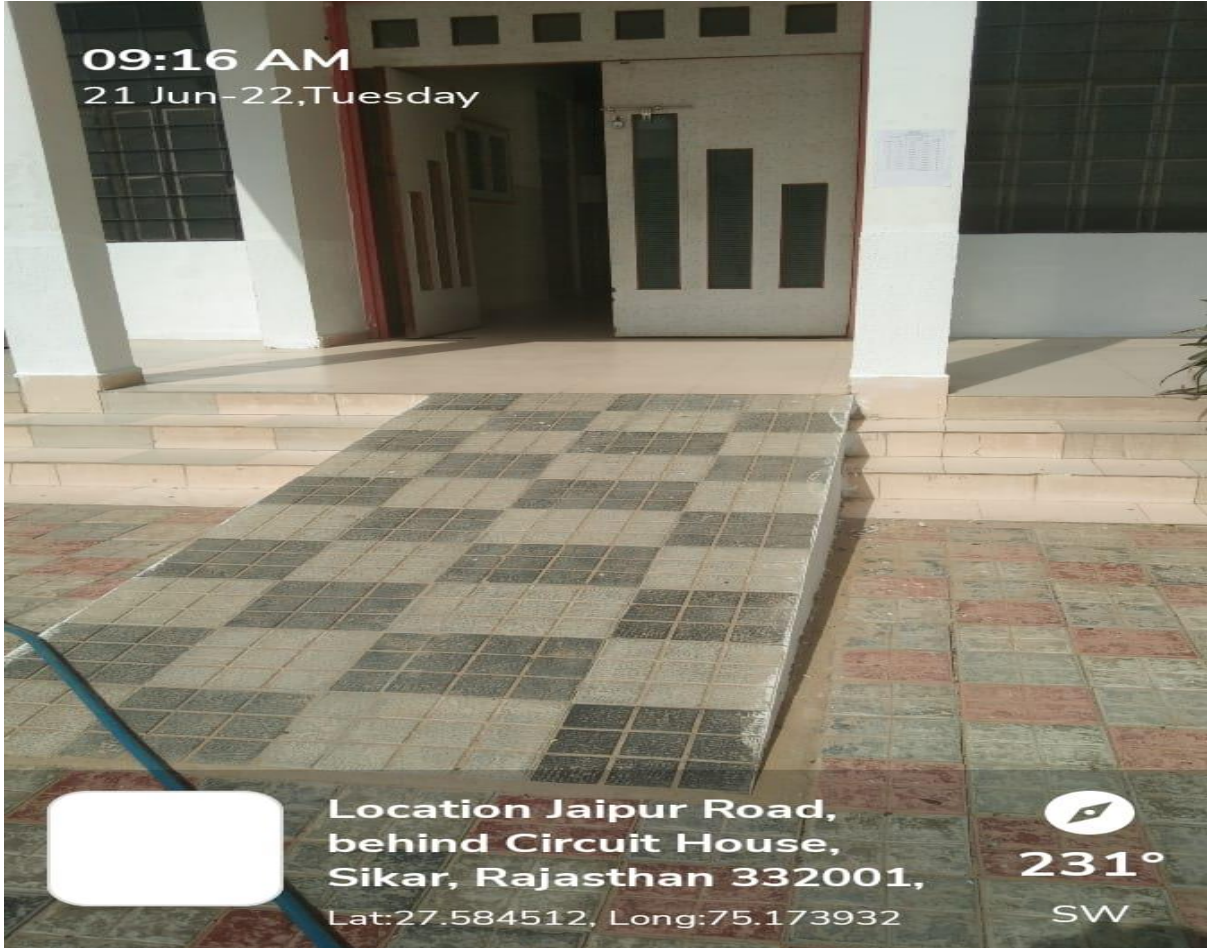
Ramp for Divyangjan
